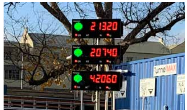
High-visibility LED displays allow truck drivers to know their axle and gross vehicle weights without needing to stop and retrieve a ticket or interact with a scale attendant.
